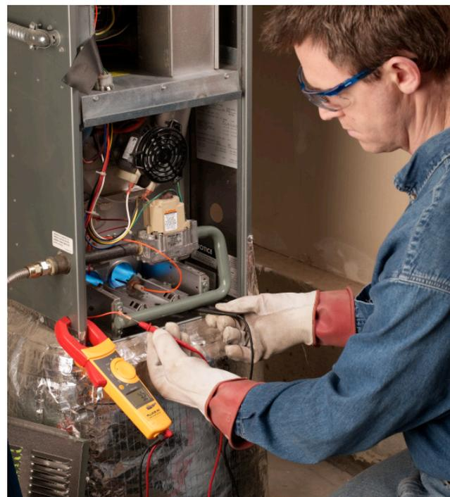
Testing the flame rectification circuit on a residential furnace.
