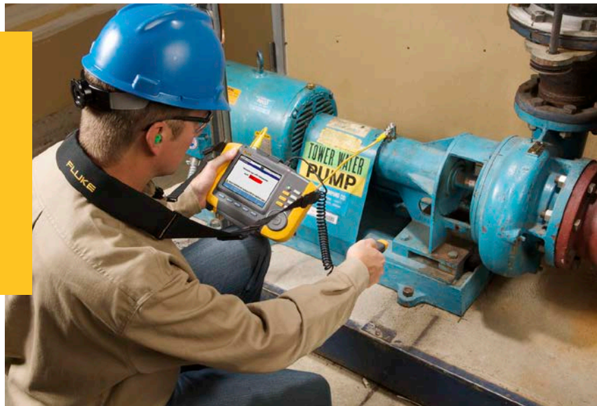
Understanding vibration analysis can change a “run to failure” system to a condition-based, proactive maintenance program.
