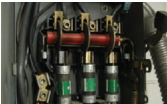
Figure 6: Power disconnect with knife blade connectors.
