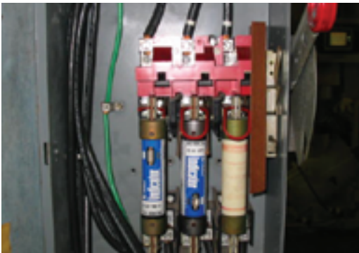
Figure 1: Fused power disconnect.
